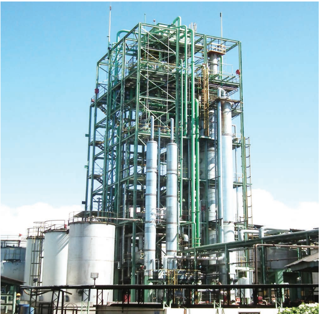
SUPPORTING SUSTAINABLE SOCIO-ECONOMIC DEVELOPMENT : A Distillation Tower at Ethanol Company Limited, Dwangwa.
